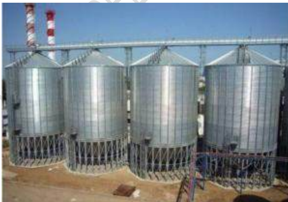
Fig. 2. Metal silos with conical bottoms for sunflower storage
